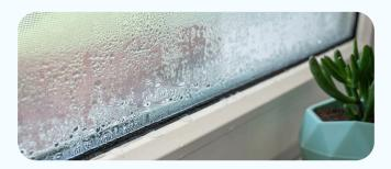
Condensation is normally found on cold surfaces such as walls, windows/window sills or mirrors, and is more prominent in the colder months. The most common signs of condensation is water collecting on windows, or black mould which can appear on any walls of the property.
