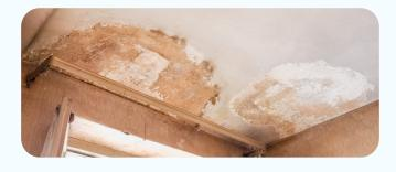
Damp occurs when a fault in the building's basic structure lets water in from the outside, and can penetrate walls, floors, and ceilings. You may see damp patches or tide marks on the walls, or peeling paint or wallpaper.
